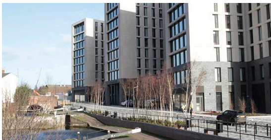
Figure 1: Photo of the Outside of University Locks
